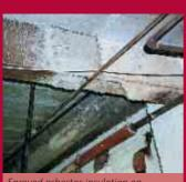
Sprayed asbestos insulation on steel framework
