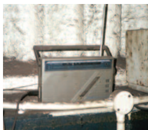
Sprayed coatings on wall
