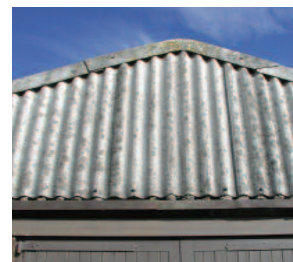
Asbestos cement panels
